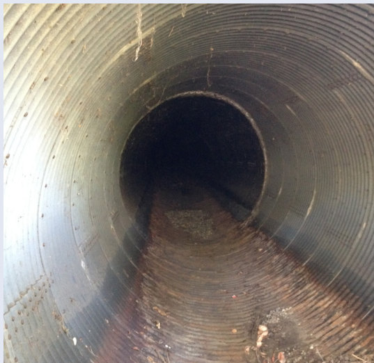
A typical corrugated steel pipe (CSP) culvert during a dry season.
